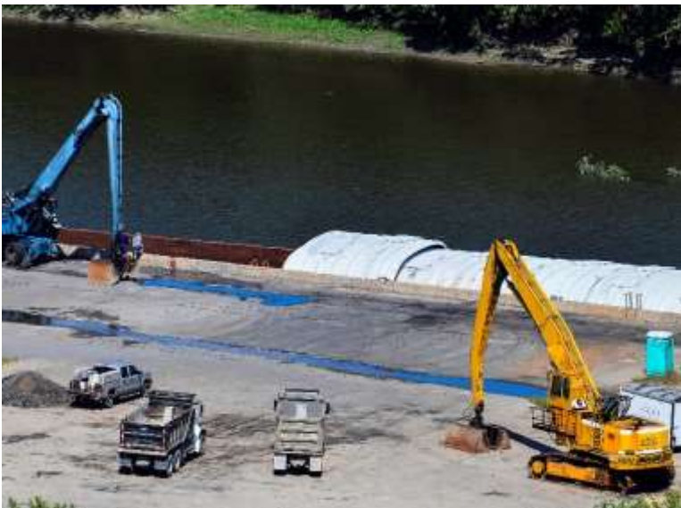
CD Terminal Operating at the Port's Little River Bulkhead
